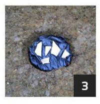
Finally wrap the membrane over the top of the hardcore/ shingle/scalpings and lay some slabs on top to seal the top. You now have a very effective soak-away.
